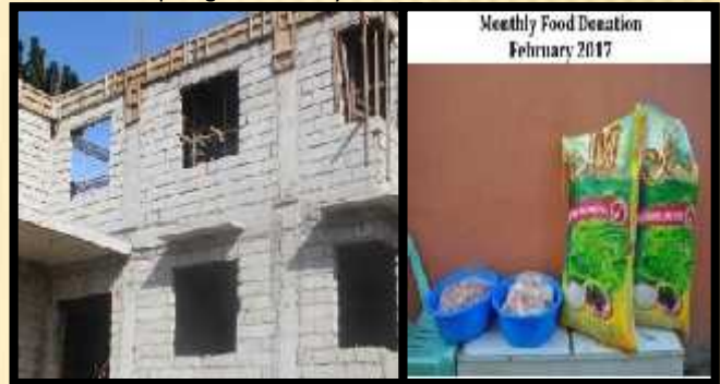
ZC Makati Central Business District - TAHANAN STA. LUISA – is finishing the construction of the Tahanan Sta. Lucia (TSL), a crisis Intervention Center. They help rebuild the lives of abused girls & they provide their daily meals.
